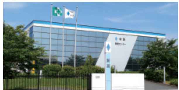
Development center to develop cleaning technology and perform analysis
